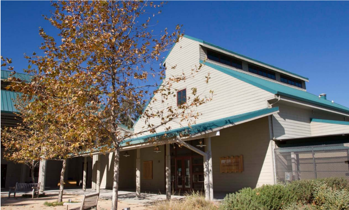
Figure 2-10 Looking West at the Entrance of the OC Agricultural and Hikkei Heritage Museum
