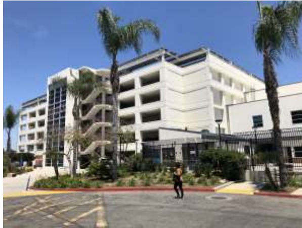
Photograph 8. View of the onsite Student Rec Center, facing northwest.
