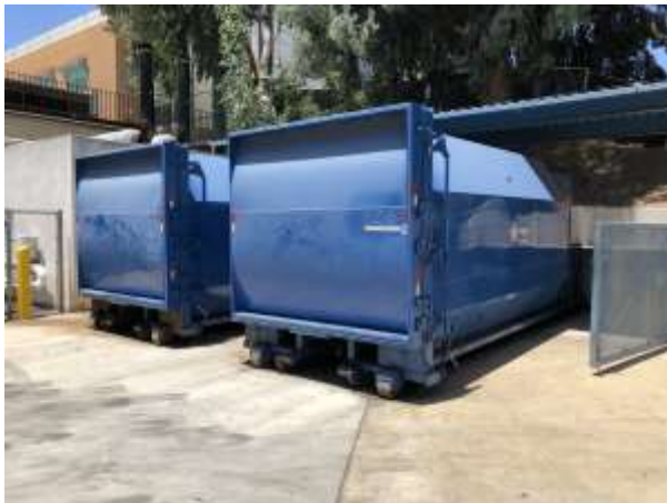
Photograph 34. Two trash compactors at the library loading dock.
