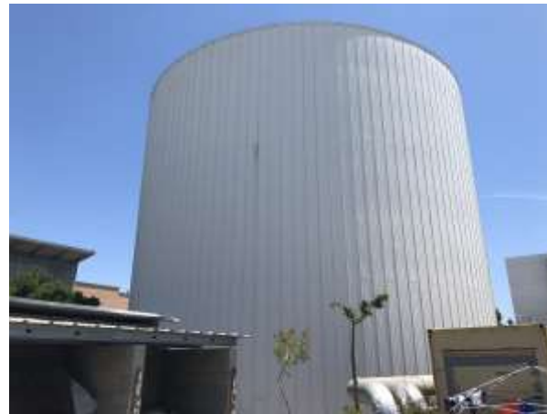
Photograph 23. View of the exterior of the chilling room.
