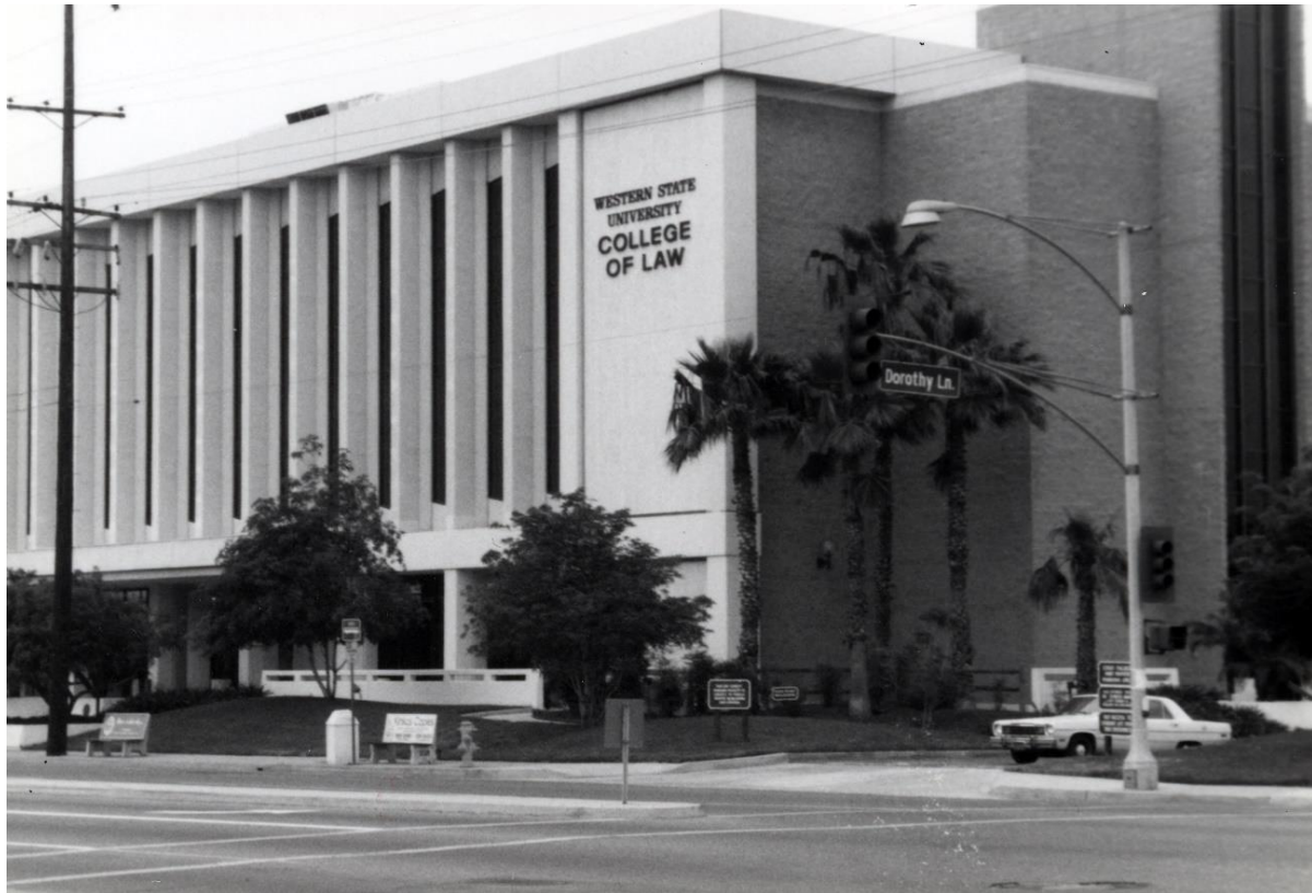
Figure 40 View of Titan Hall, Previously Part of Western State University College of Law
