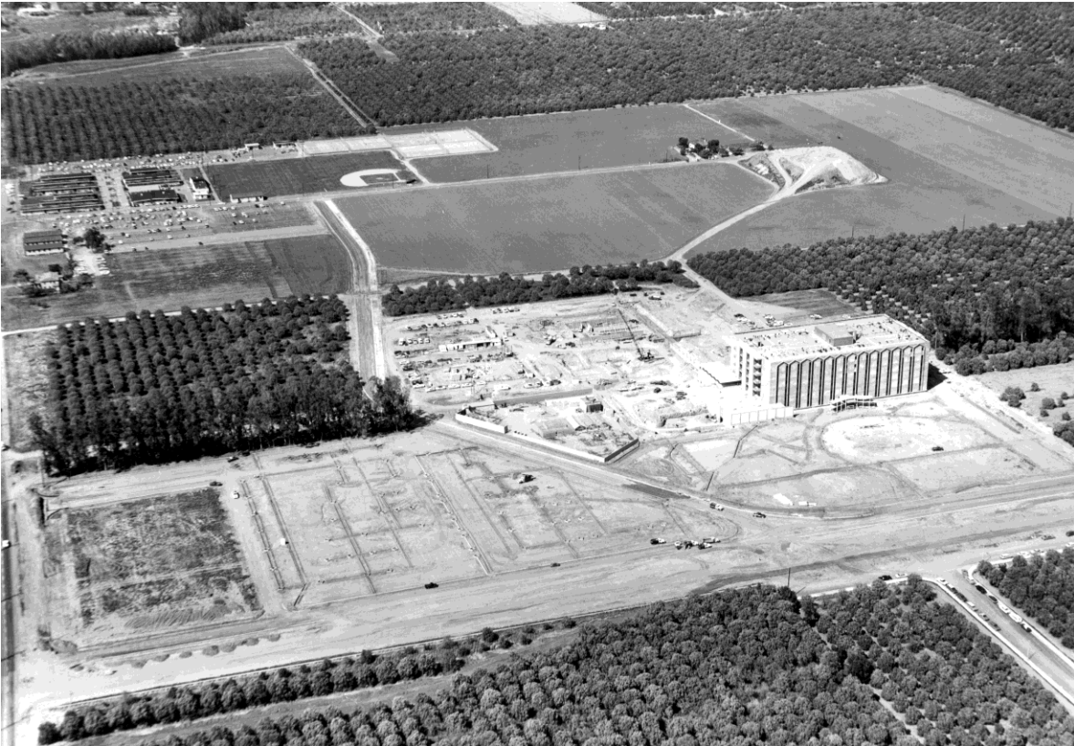
Figure 22 Aerial Showing Construction of Letters and Science Building
