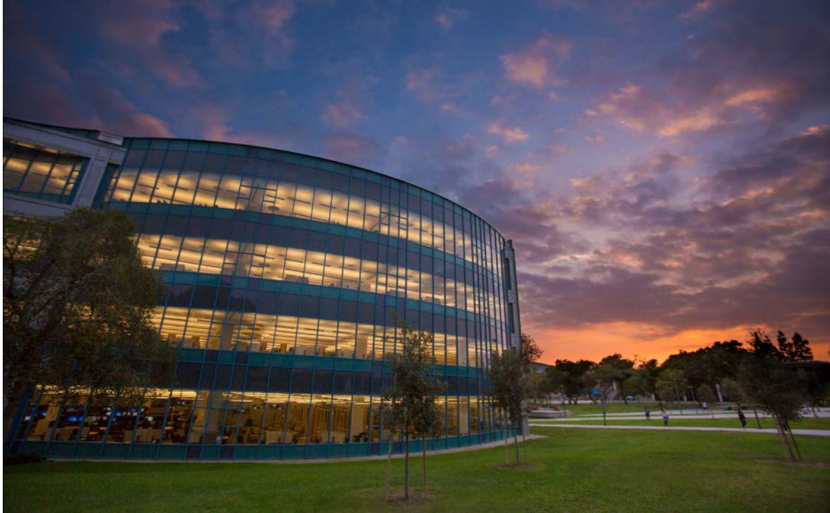
Figure 2-16 Looking Southwest at Pollak Library
