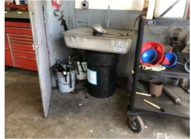
Photograph 3. View of the parts washer at the Facilities and Maintenance Auto Shop.
