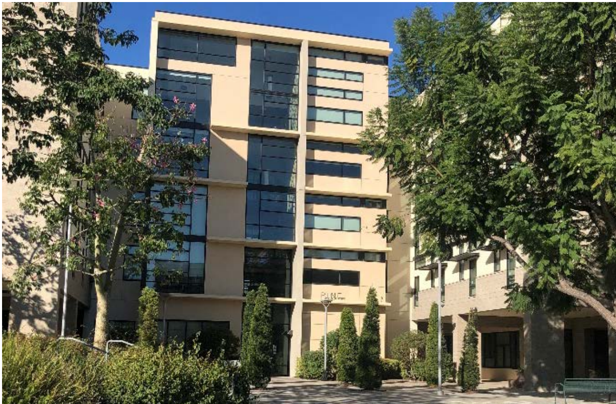
Figure 2-19 Looking North Towards Juniper Residence Hall
