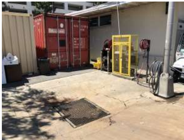
Photograph 5. View of the onsite wash area and pump near the Receiving buildings.
