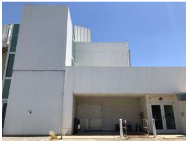
Photograph 29. View of the exterior of the DBH building.
